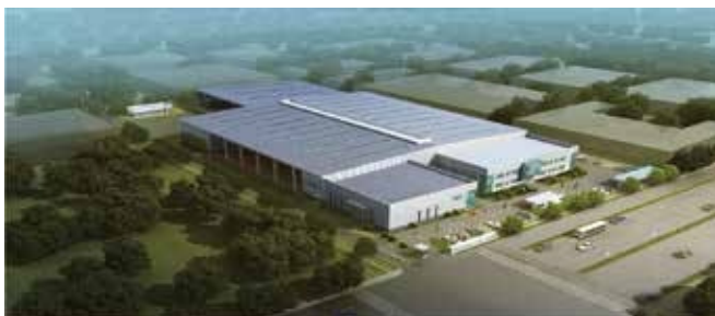
Oil injected screw compressors and Refrigerated Dryer plant: Pan-Asia, Wuxi
